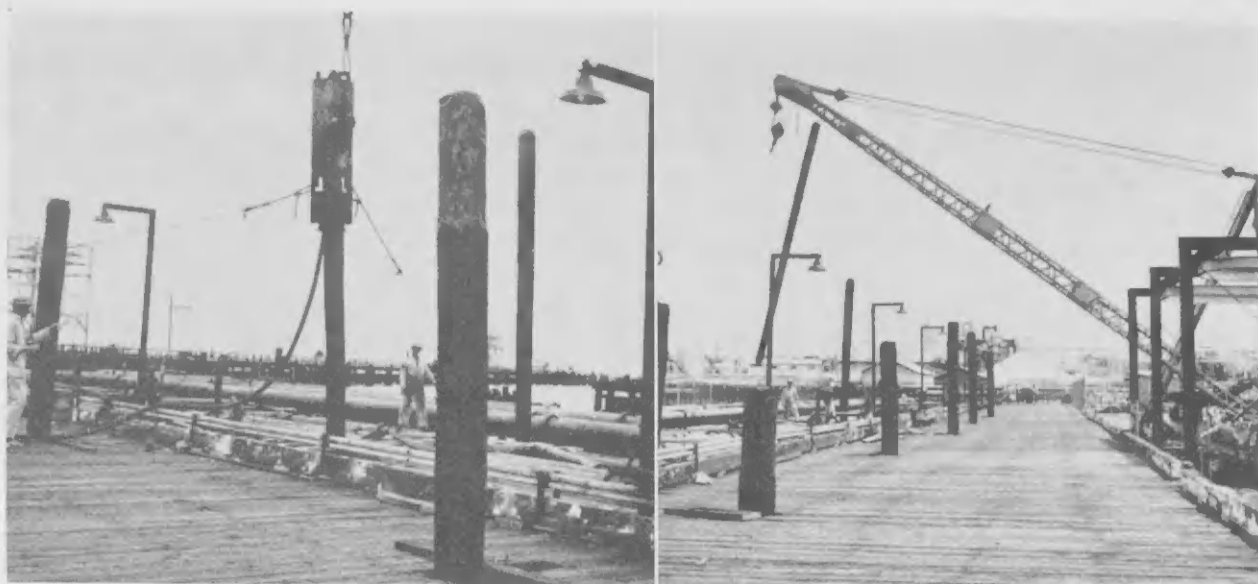
THE TRESTLE that once supported the rails for sulphur carrying carts will soon be dismantled. It will be replaced by a six-foot-wide walkway to the Gasoline Docks. Until 1954, Lago imported its sulphur requirements from Louisiana.
